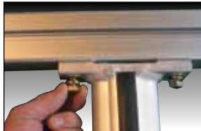
6B hand tight 16 bolts before wrenching
