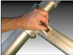
9B T-Bolts inserted
